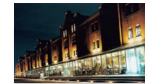
Yokohama Red Brick Warehouse Warehouse No. 2 (2002)
